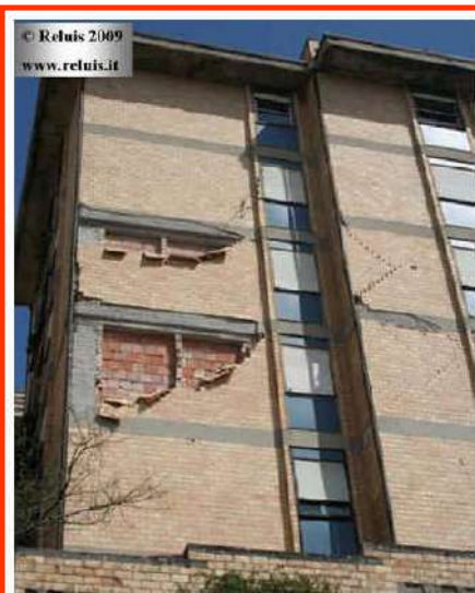
Infills damage Internal infill is made up of clay blocks, external one of solid bricks.
