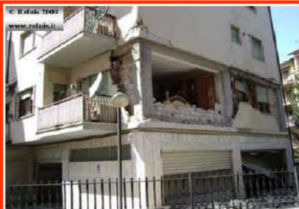
Reinforced concrete building placed in Via XX Settembre – L'Aquila Total and partial ejecting of corner infills at first level.
