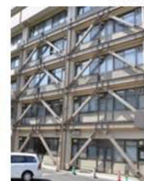
Applied Chemistry and Chemical Engineering Building (Sendai, Giappone)
