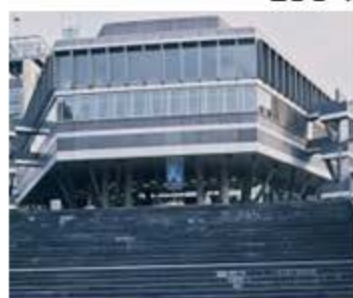
Auditorium HPH oh ETH (Zurich, Switzerland)
