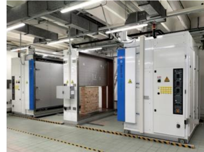
Camera termica - Sustainable Energy Laboratory (DICAM UniTN)
