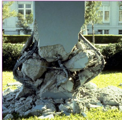
Photo 1.1 Ductile concrete, Northridge earthquake, 1994. (Courtesy of Englekirk Partners, Inc.)
