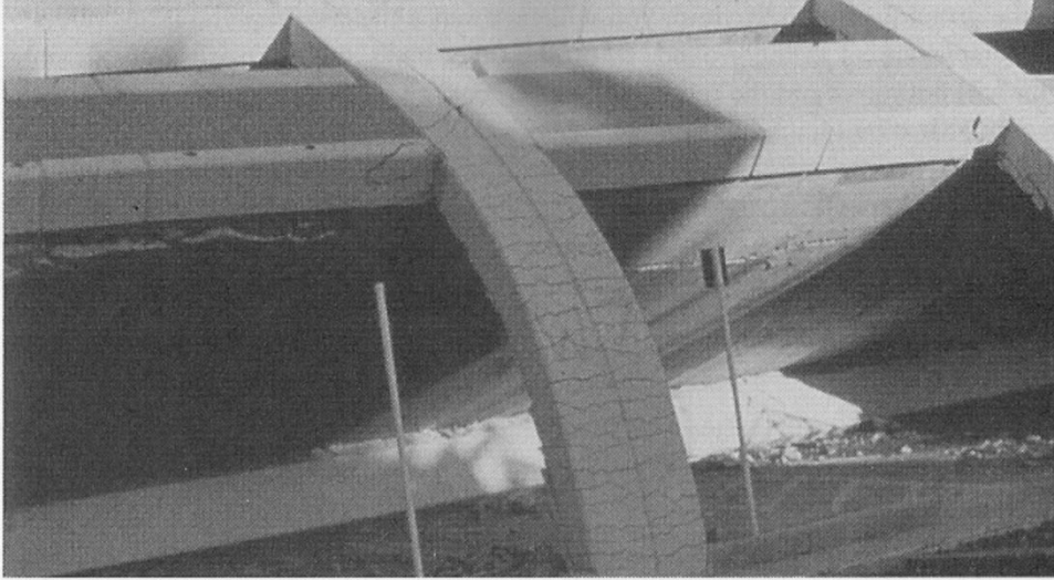
Photo 1.1 Ductile concrete, Northridge earthquake, 1994. (Courtesy of Englekirk Partners, Inc.)
